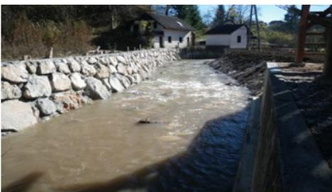
Picture 13: Example of widening and straightening the riverbed with the concrete stabilization of river banks. Photo: FRIS.
